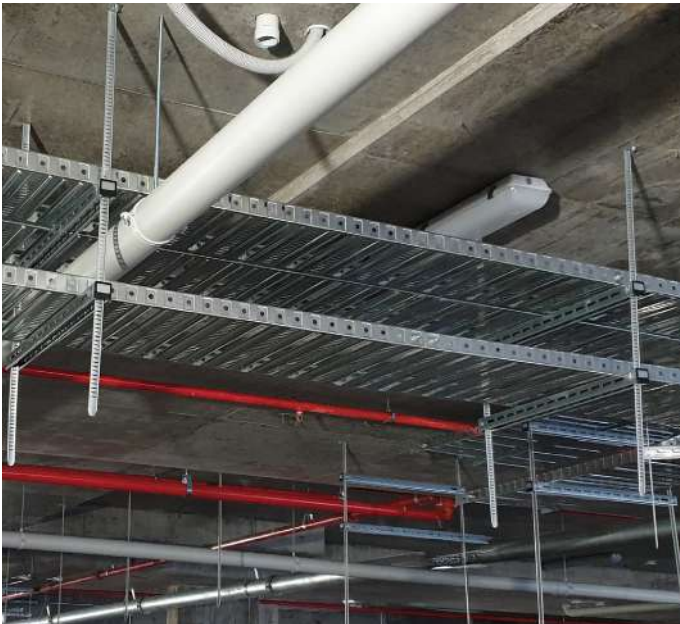
Installation of Double Stack Cable Tray
