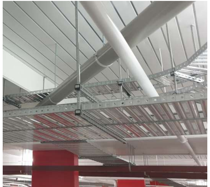
Installation of Side by Side Cable Tray
