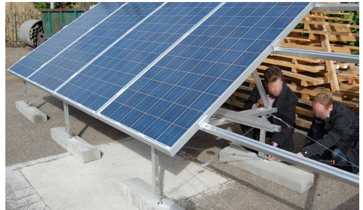
Solar Panel Installation
